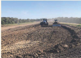
Raising a levee with new fill.
